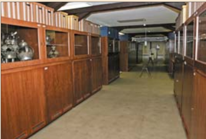
As part of building work in the Maisel Synagogue, alterations were carried out in order to provide a more effective use of non-exhibition spaces. The loft space was extended to produce a depository of synagogue textiles and metal artefacts. Depicted is the newly constructed depository which is intended for the Museum's rarest synagogue textiles.
